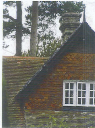
Picture 9.17 Gable ends
