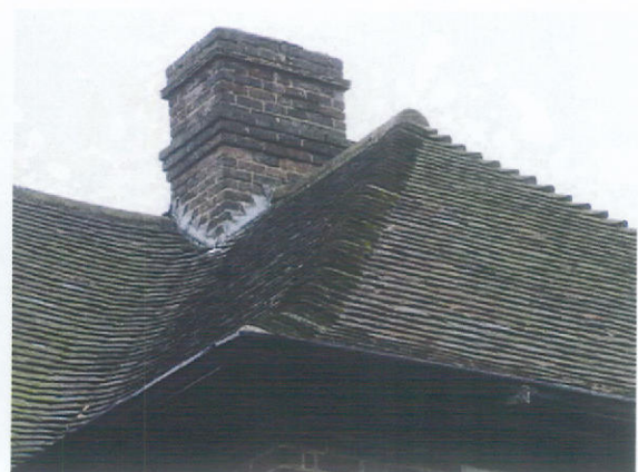
Picture 9.20 Tiled roofs
