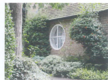
Picture 9.30 Oval windows
