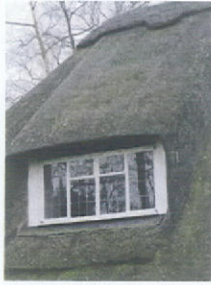
Picture 9.31 Thatch roof
