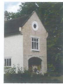
Picture 9.27 Stone lintels
