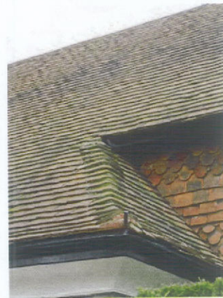
Picture 9.38 Deep red clay tiles
