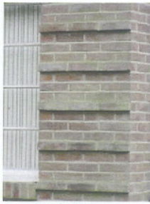
Picture 9.25 Projecting bricks
