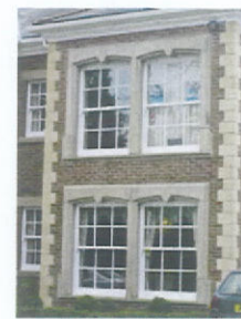
Picture 9.36 Stone quoins and window surrounds
