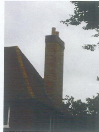
Picture 9.18 Tall chimneys
